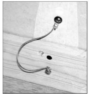
**SAFETY CABLE** This screw, when properly driven into the stud, should be fairly hard to drive. If it is not, you may have missed the stud and should try again. *The function of this cable is to make attachment failure of the bed visible by allowing it to come away from the wall. two or three inches. When you see this condition DO NOT OPEN THE BED! You **must** investigate what is wrong and correct it!*
